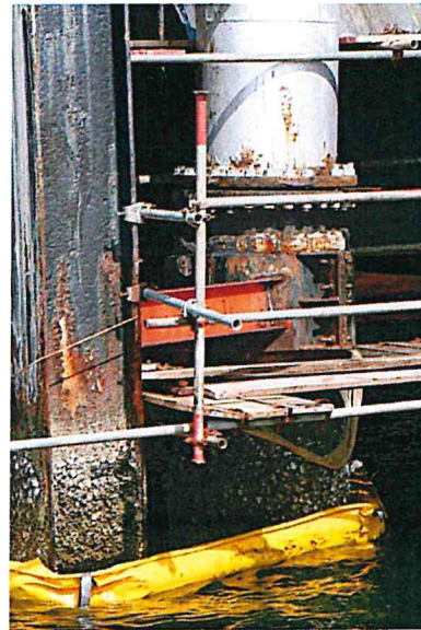
Figure B-9 Sea Line 36 at Berth 5.
