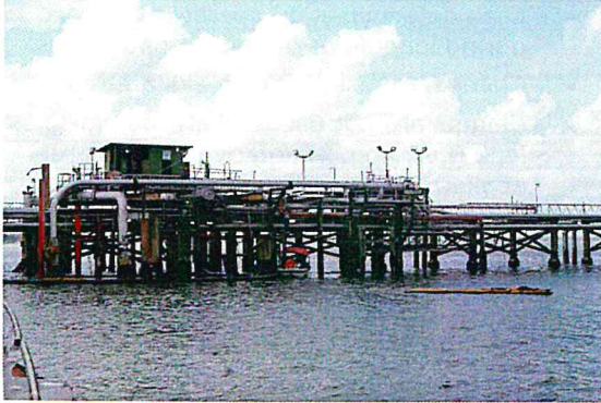
Figure B-2. Main pipe viaduct near Pile Bent (PB) 80.
