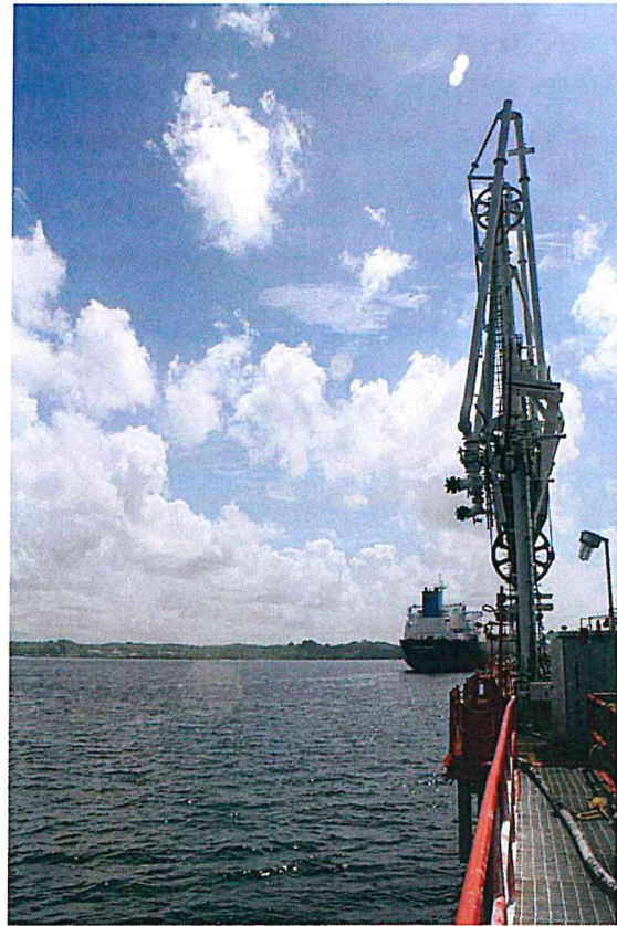
Figure B-16. Loading arms at Berth 6.
