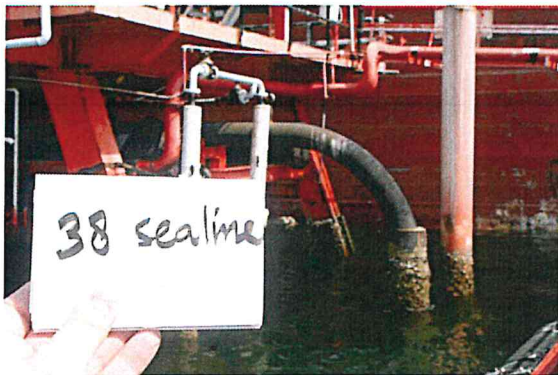
Figure B-7 Sea Line 38 at Berth 5.
