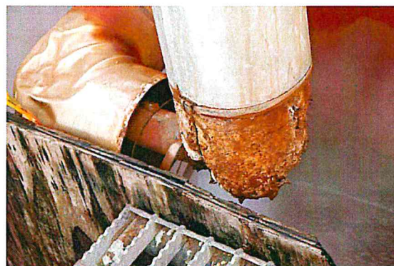
Figure B-73. Close up view of previous photograph.
