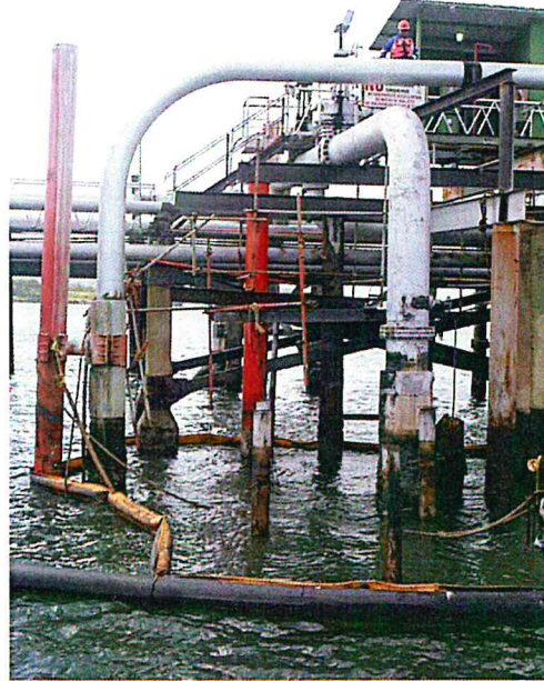
Figure B-4. Close-up view of repair work near PB80.
