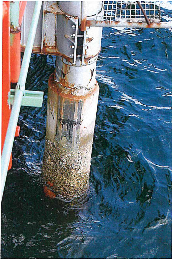
Figure B-15. Sea Line 38 (out-of-service) at Berth 6.
