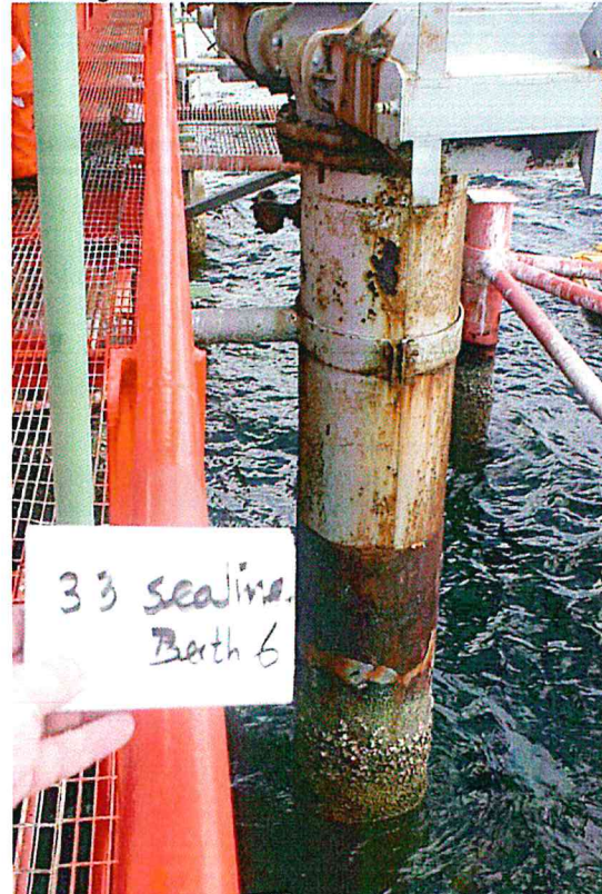
Figure B-14. Sea Line 33 at Berth 6.
