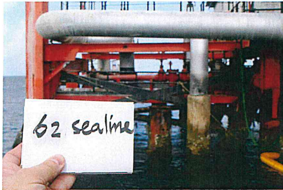
Figure B-6 Sea Line 62 at Berth 5.
