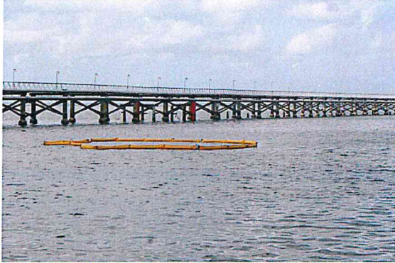
Figure B-1 Near main pipe viaduct: Boom in the water around area where Sea Line 61 Clamp was reported.
